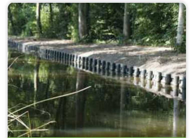
RIVER BANK PROTECTION
