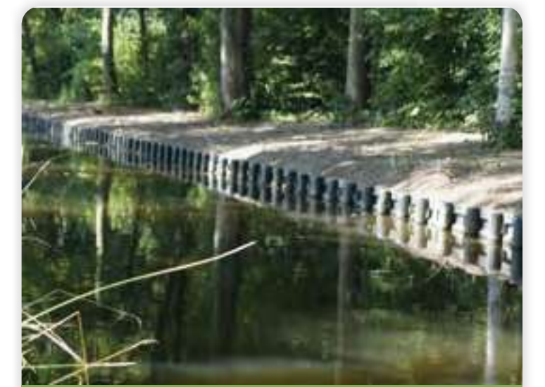
RIVER BANK PROTECTION
