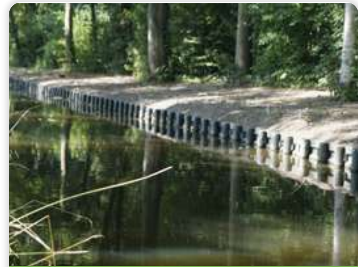
RIVER BANK PROTECTION
