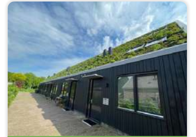
GREEN ROOF FRAME
