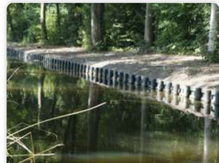
RIVER BANK PROTECTION
